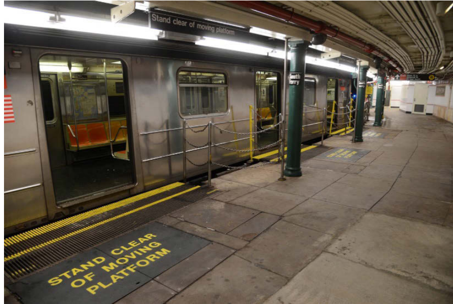
Figure 9. Moveable platform at South Ferry Station New York subway
