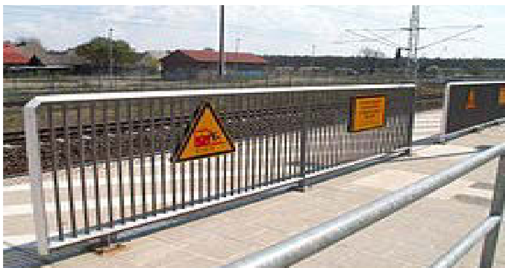
Figure 8. Platform Barrier with gates
